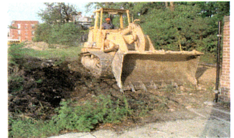
Clearing the lot
